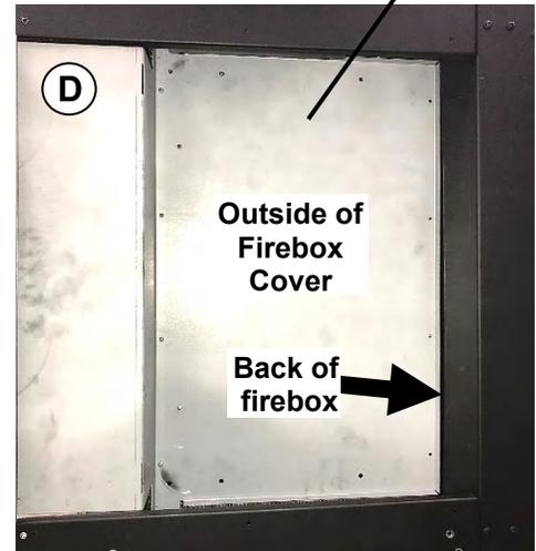
**STEP THREE: INSTALL INNER LINER PANEL**
