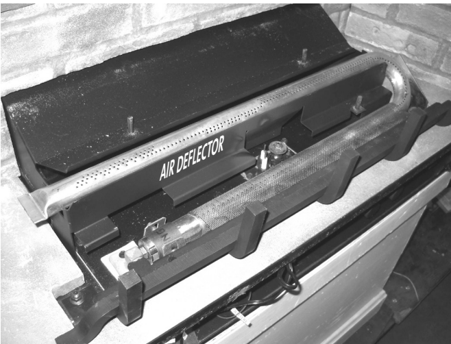
Figure 25. Correct burner tube alignment.
