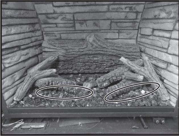
Figure 86: Placement of extra large ember chunks.
