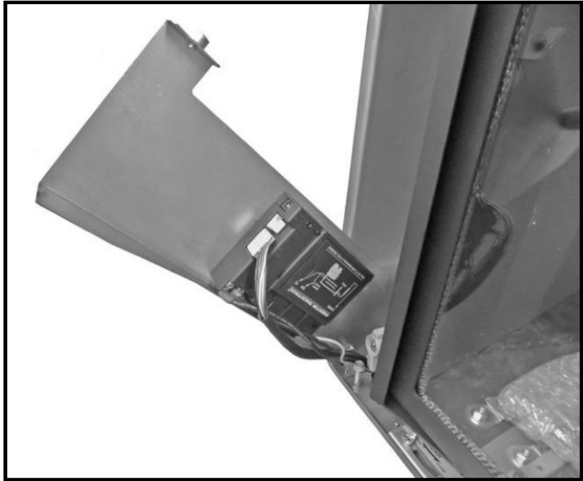
Figure 39: Maxitrol electrical controller in its caddy.
