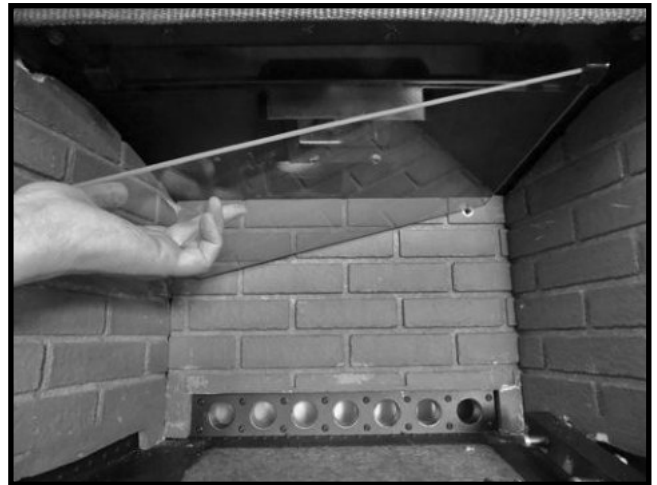
Figure 31: Inserting baffle into the upper corner.
