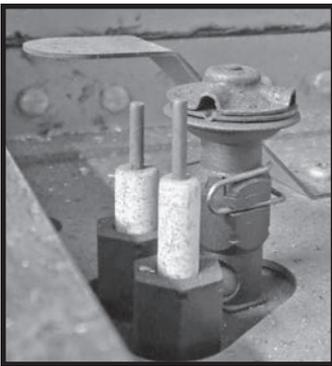
Figure 70: Trenton pilot assembly.
