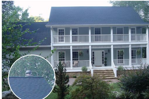
When the owners of a home in Atlanta, GA, realized their fireplace was venting into a deteriorating chimney and creating a fire hazard, they had to choose between recreating the fireplace opening—or installing a (barely) noticeable RS Chimney Fan.
